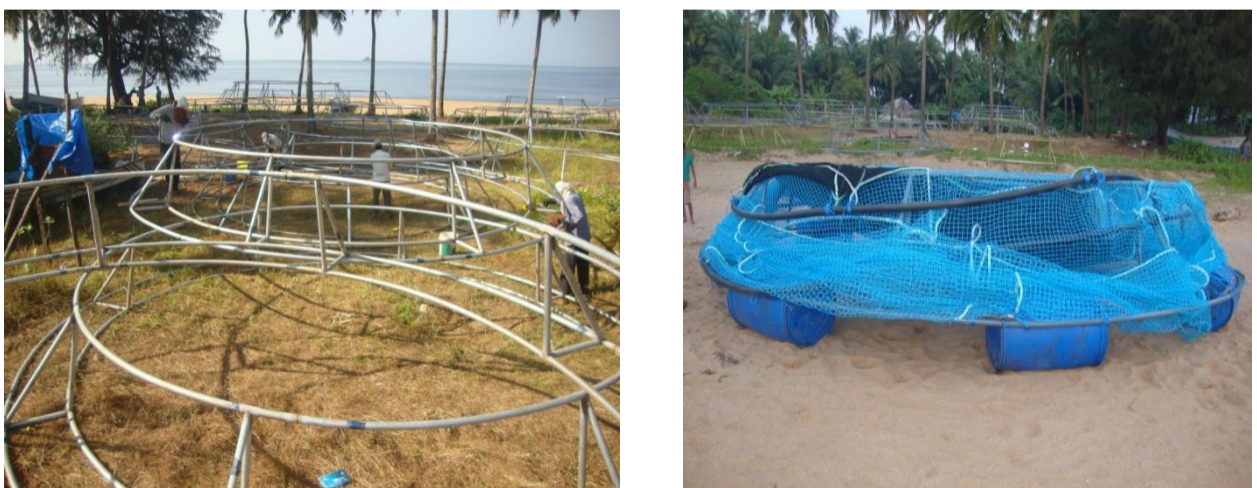
Construction of cages
