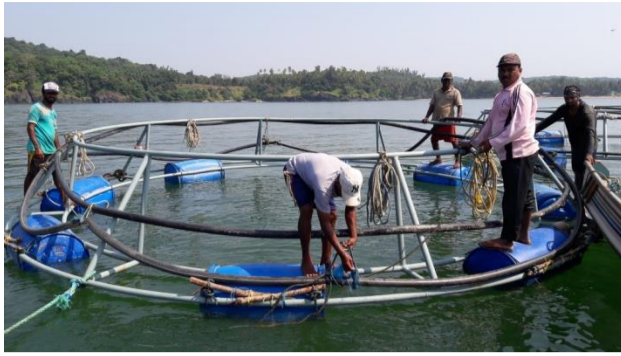
Installation of cages
